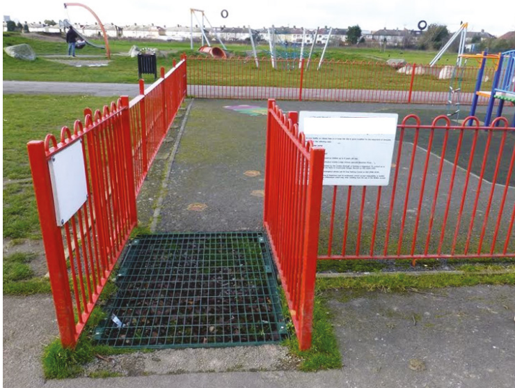
Figure 5: A dog grid installed to stop dogs entering the play area, which will impact on the accessibility of the play area to those who rely on assistance dogs.
